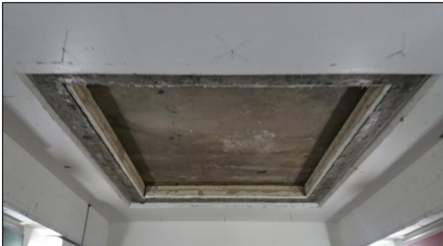
Photo No. 2 Receive Room View of Test Specimen Installation
